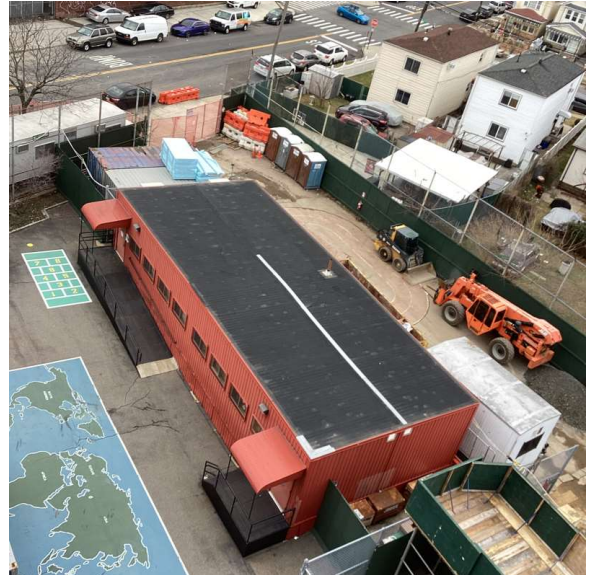
Roof 1 - Northwest view
