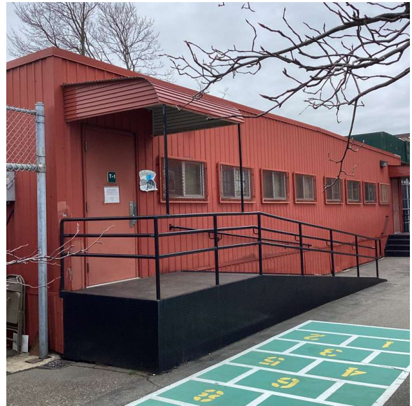
Corner of Facades B and A - Northeast view
