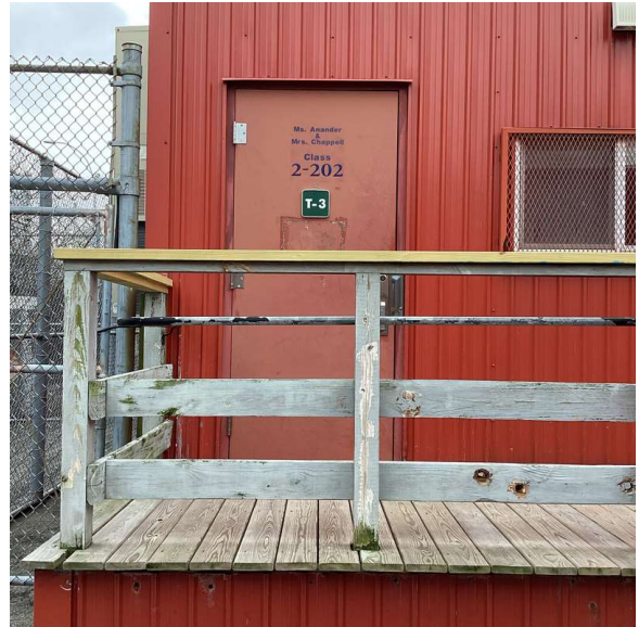
Facade E - Unit T3
