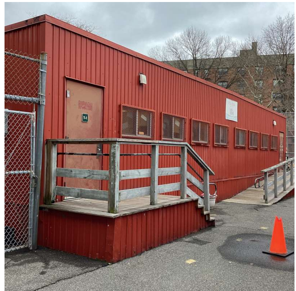
83rd Street - Northeast View
