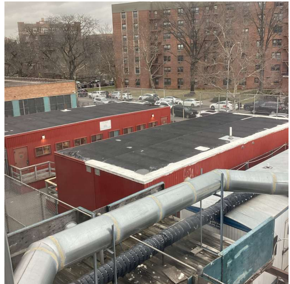
Roofs 1, 2 - Northeast View
