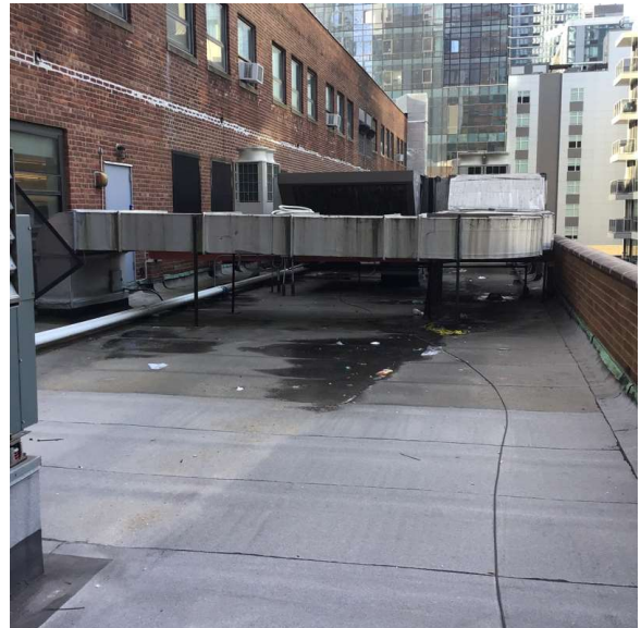
Roof 1 - Southwest view
