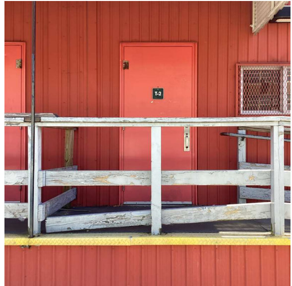
Facade A - Unit T2
