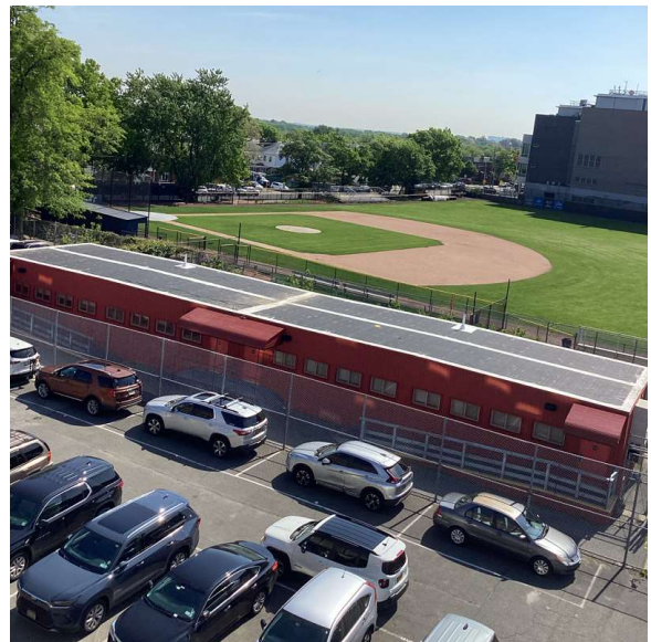
Roof 1 - South View
