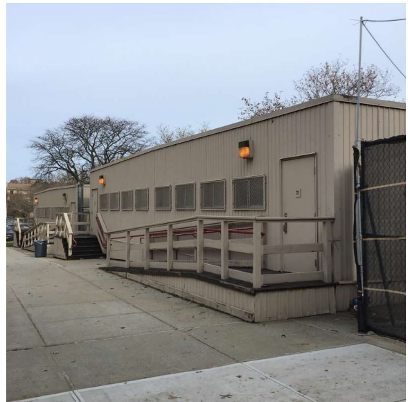
Corner of Facade A and D - North View
