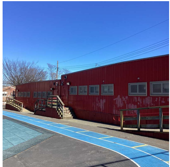
Facade A - Northeast view
