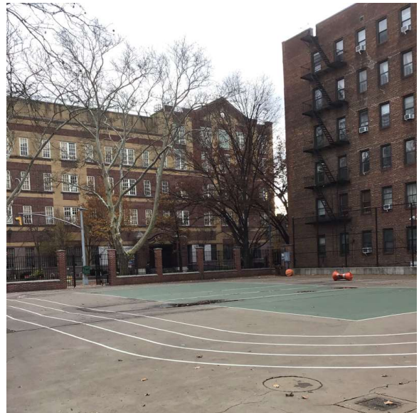
Play yard - Southwest View
