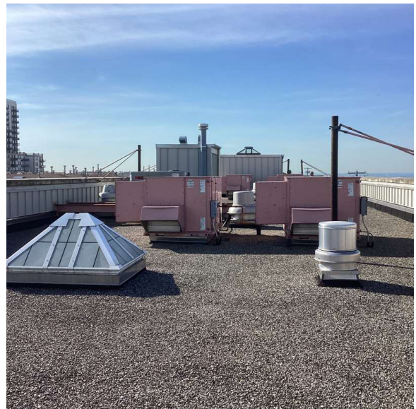
Roof 1 - South view
