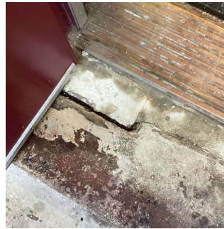
Facade B No violations recorded.
