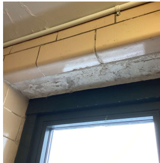
Roof 1 - Bulkhead No violations recorded.
