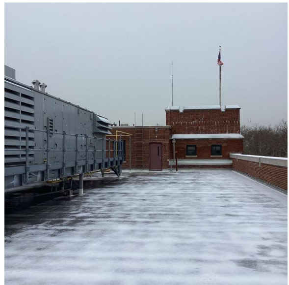
Roof 1 - Southwest view
