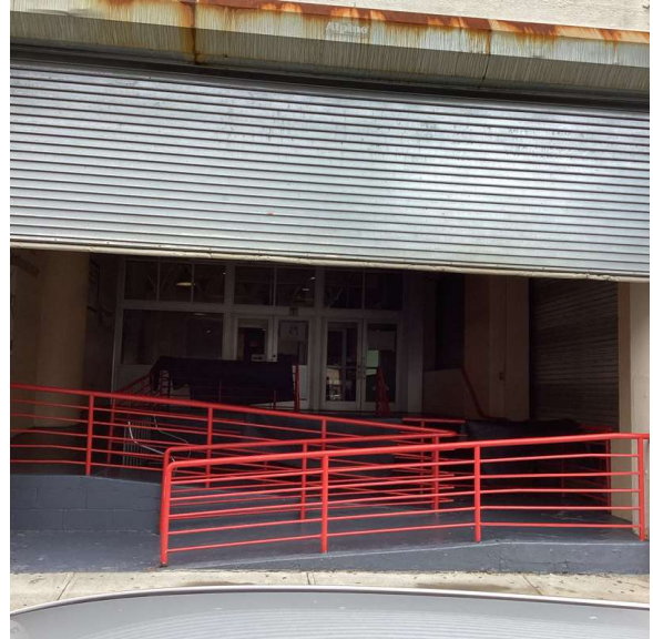
Facade A - 30th Place
