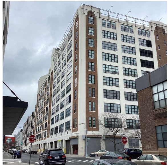
Corner of 48th Avenue and 30th Place - Northeast View
