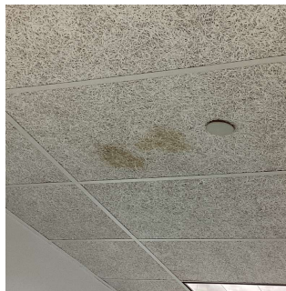
Roof 1 - 2nd Floor Corridor near Room 223
