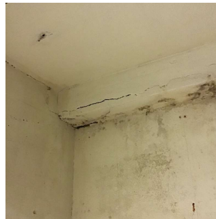
Basement - Oil Tank Room
