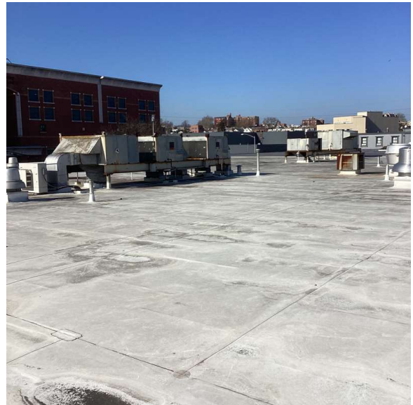
Roof 1 - Northwest View
