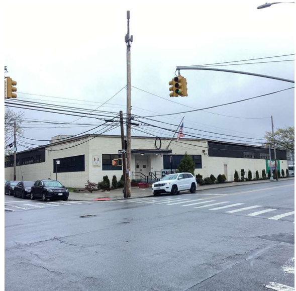
Corner of 51st Avenue and Jacobus Street - Northeast View
