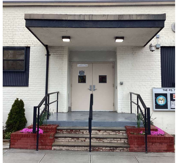
Facade A - 51st Avenue
