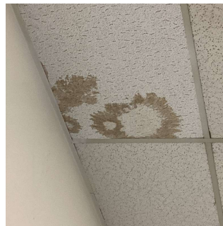
Roof 1 - Cafeteria (three locations) also Kitchen, Rooms R118, S119
