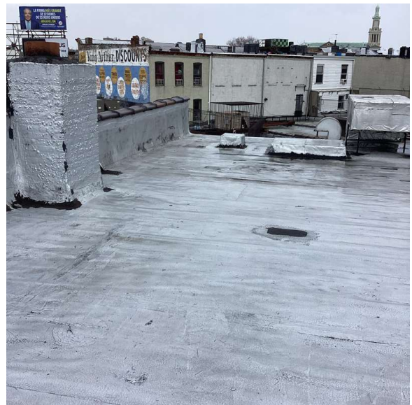
Roof 1 - Northeast View
