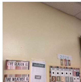
Facade E - Room 107
