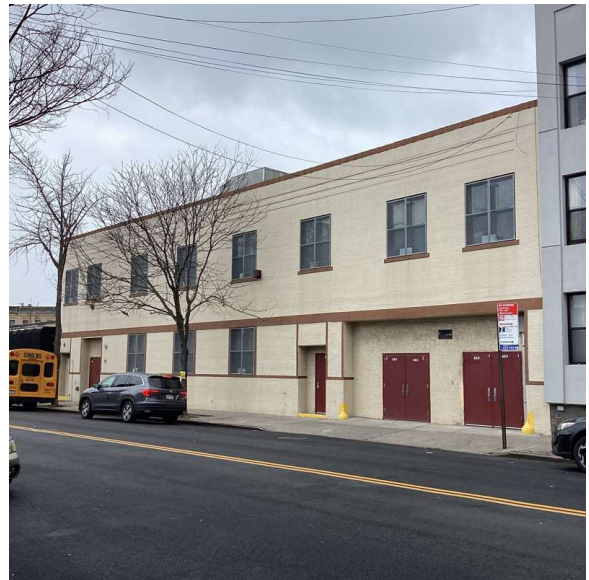
Cypress Avenue - North View
