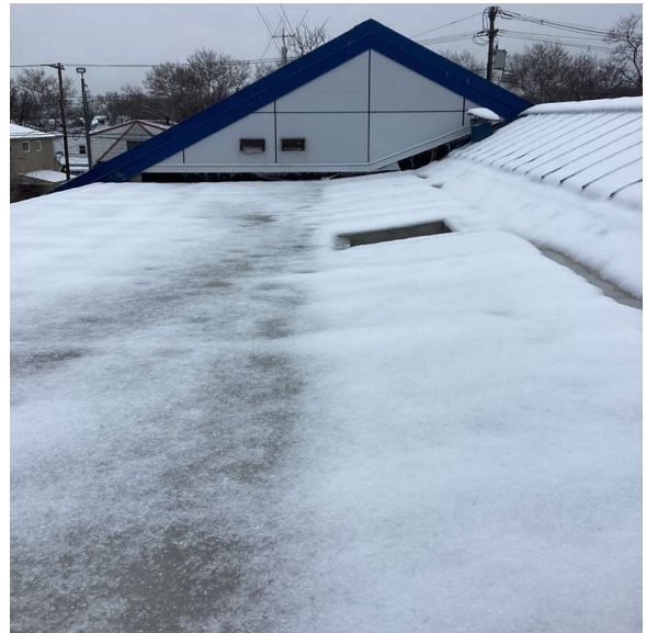
Roof 10 - South view
