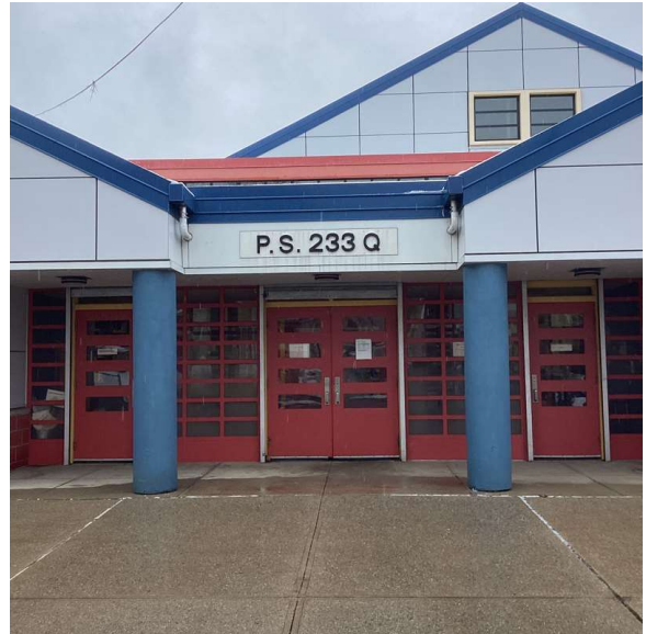
Facade A - 142nd Street
