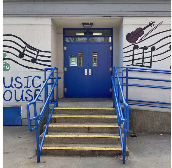
Facade A - 78th Street
