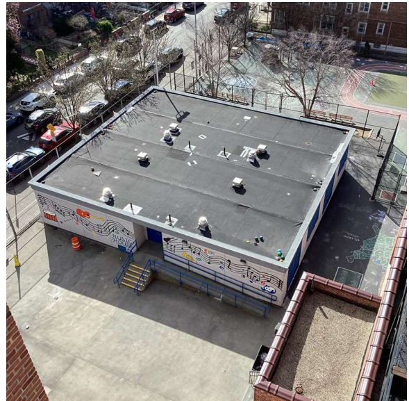
Roof 1 - Southeast View
