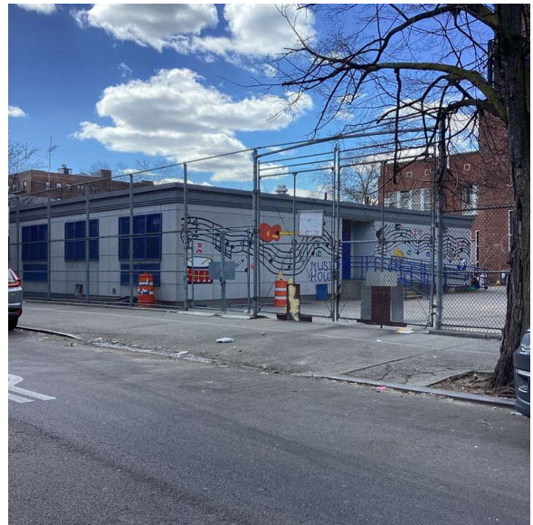
78th Street - Southwest View
