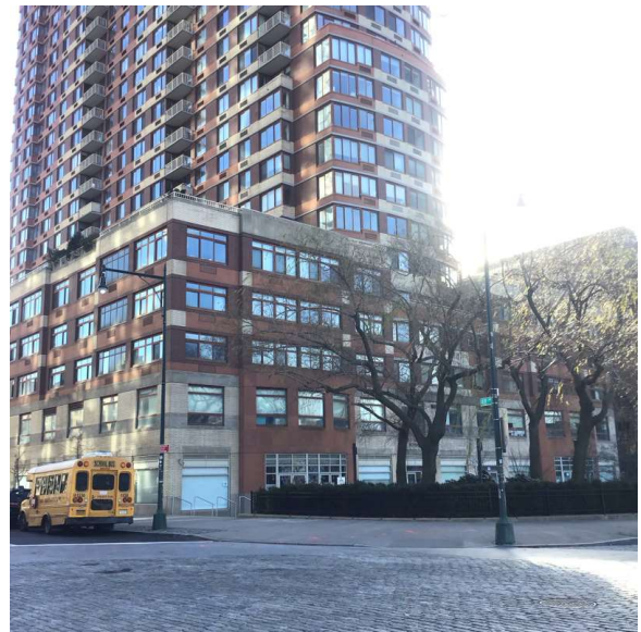
Corner of Central Boulevard and 48th Avenue - East View
