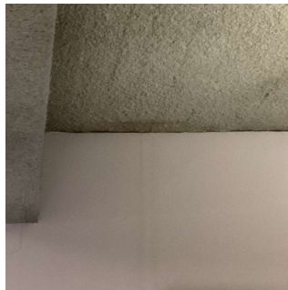
Roof 1 - Room 211 No violations recorded.
