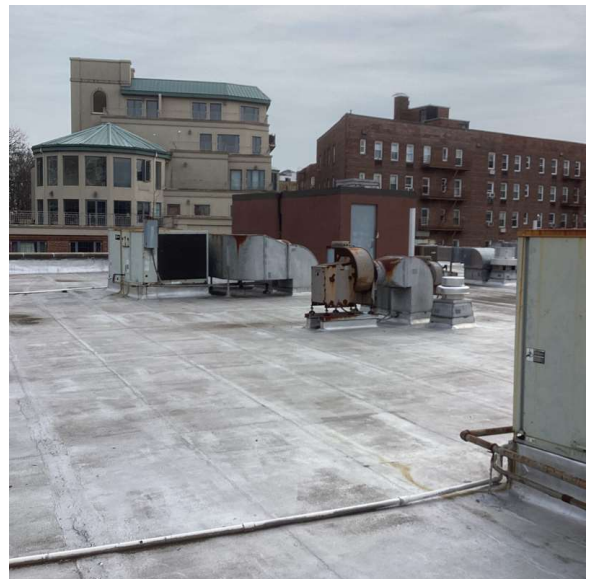
Roof 1 - South View
