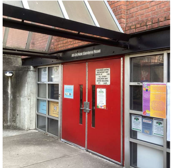
Facade A - Lefferts Boulevard
