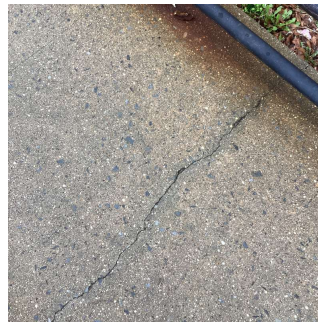
Facade C No violations recorded.
