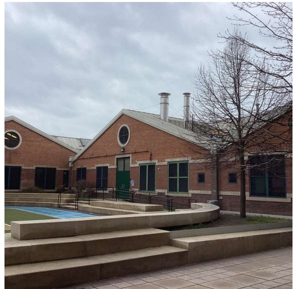
Facade A - Southwest view
