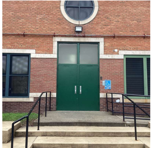
Facade A - 132nd Street
