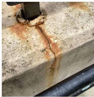
Facade A No violations recorded.
