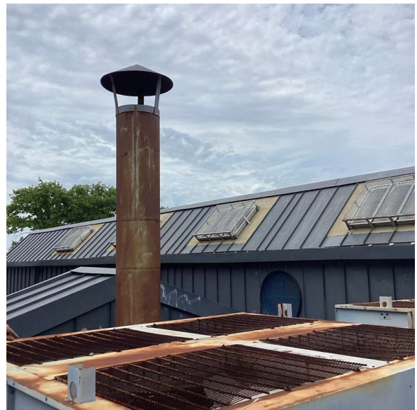
Roof 1 - Southwest View
