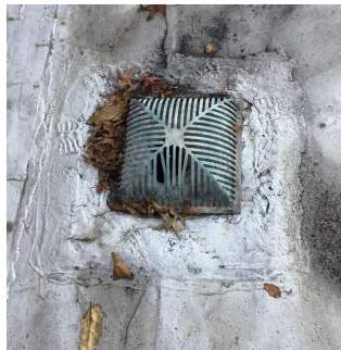
Roof 1 No violations recorded.
