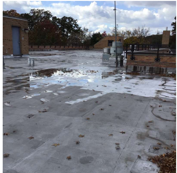
Roof 1 - West View
