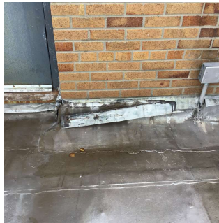
Roof 1 No violations recorded.
