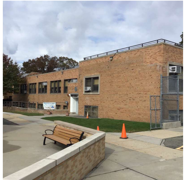
Union Turnpike - Northwest View
