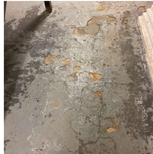
Basement - outside Oil Tank Room
