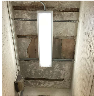
Basement - Stairs to Exit 17
