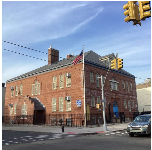
Corner of Seneca Avenue and Bleecker Street - North view
