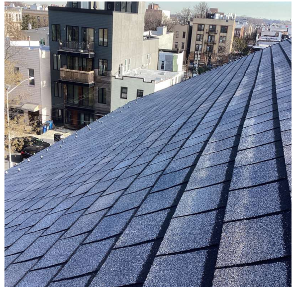
Roof 1 - Southeast view
