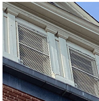
Facade A No violations recorded.
