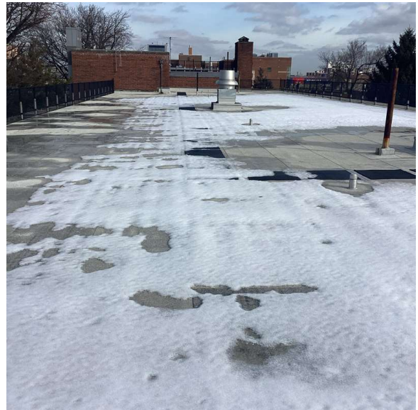
Roof 1 - Northeast View
