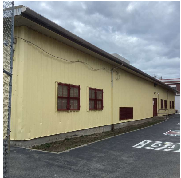
Facades A and B - Northeast view
