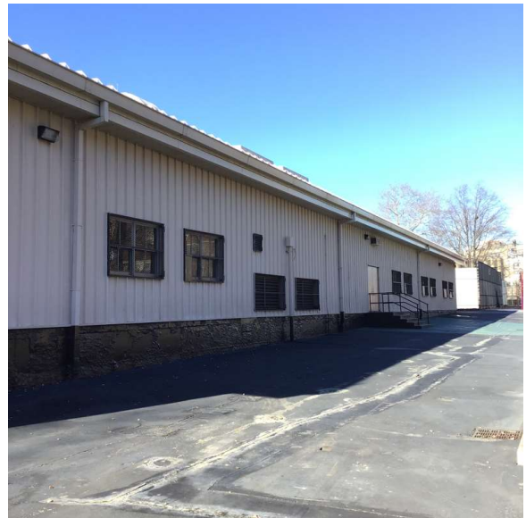
Facade A - Northwest view
