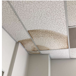
Roof 2 - Room 201, also Women's Toilet Room
