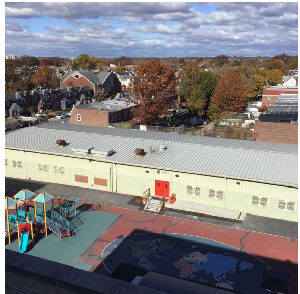
Roof 1 - Northwest view
