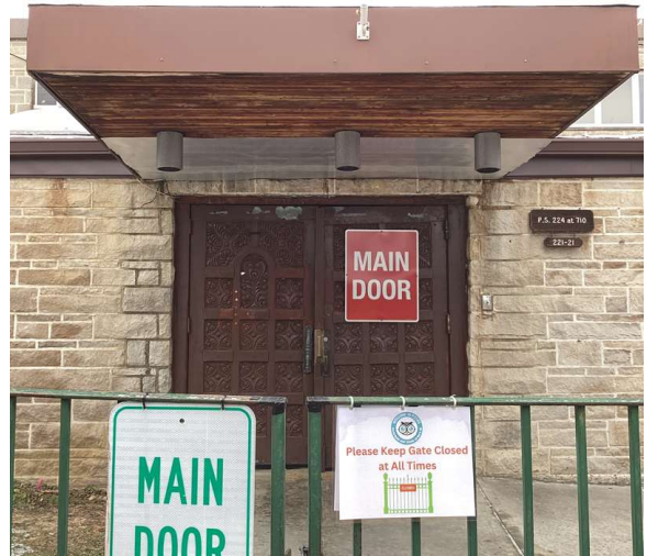
Facade A - Corbett Road
