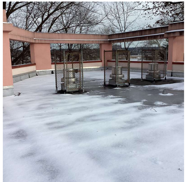
Roof 3 - East View
