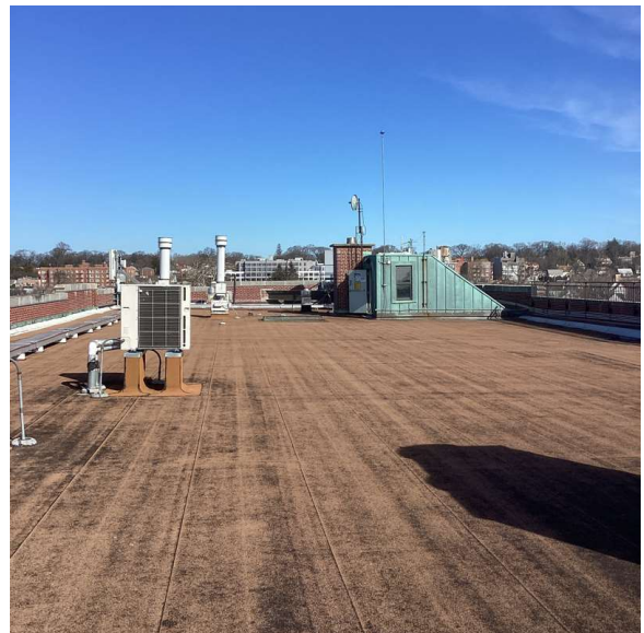
Roof 1 - North view
