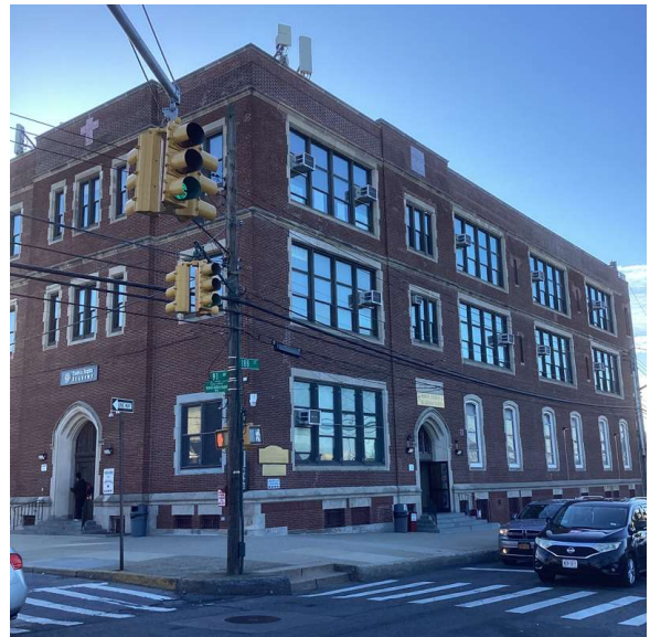
Corner of 91st Avenue and 188th Street - Southeast view
