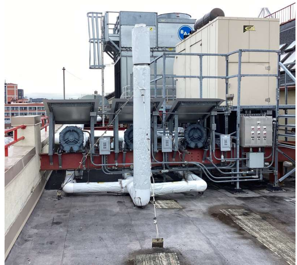
Roof 1 - South View
