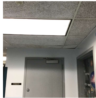
Corridor near Room 208
