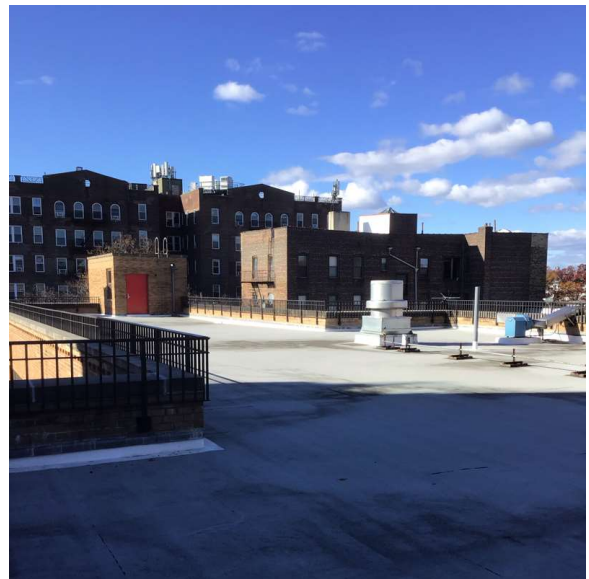
Roof 1 - Southeast View
