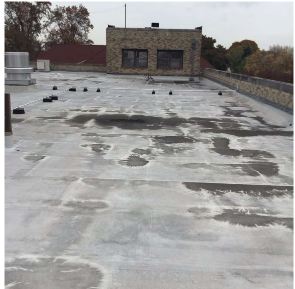
Roof 1 - Northeast View
