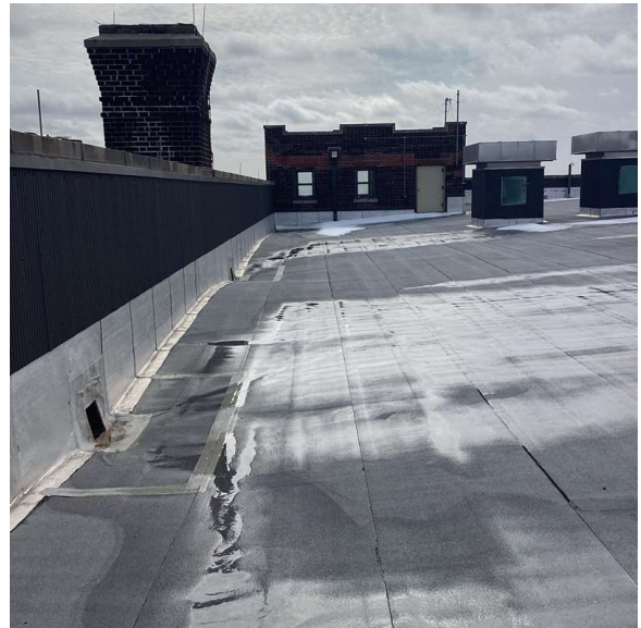
Roof 1 - South View
