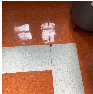
Corridor near Stair B/2
