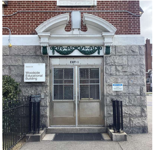
Facade A - 44th Street
