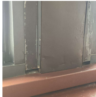
Facade B - Corridor near Room 312 No violations recorded.
