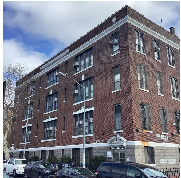
44th Street - Northeast View
