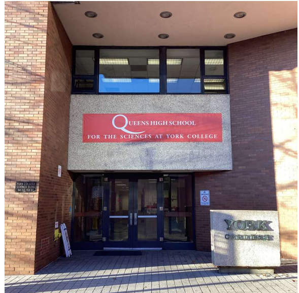
Facade A - 159th Street
