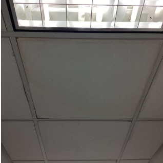
Roof 1 - Room 218, also Roof 1 - Room 222 No violations recorded.
