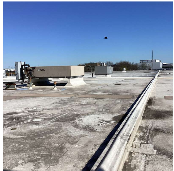
Roof 1 - North View
