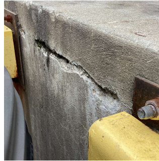
Loading Dock 1 No violations recorded.
