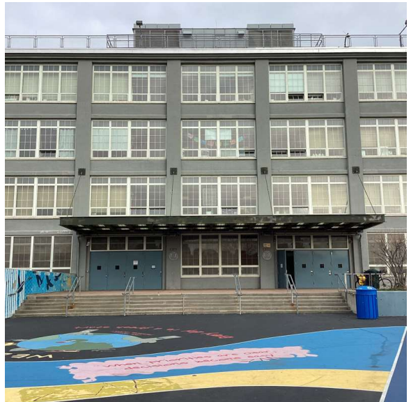
Facade A - 94th Street
