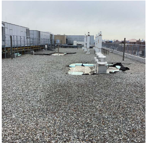
Roof 1 - Southwest View
