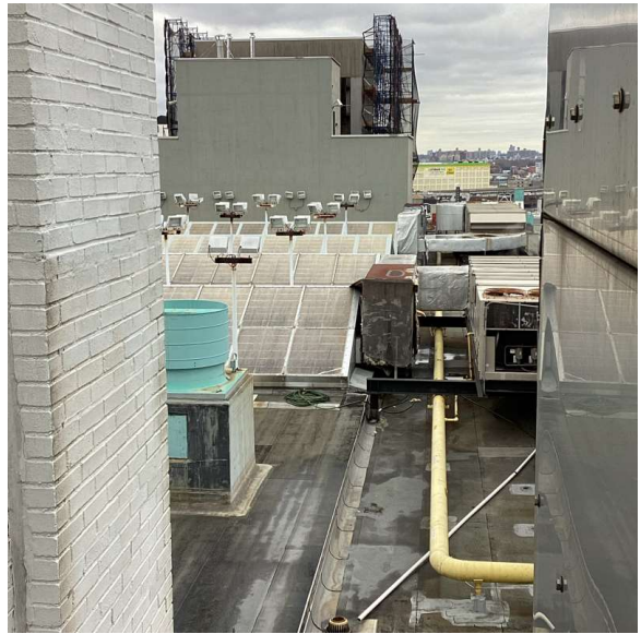
Roof 1 - Southwest View
