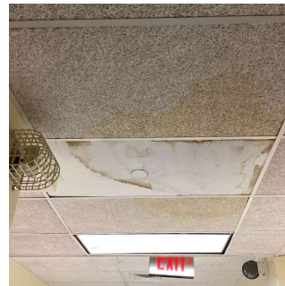
Roof 1 - Corridor near Boiler Room
