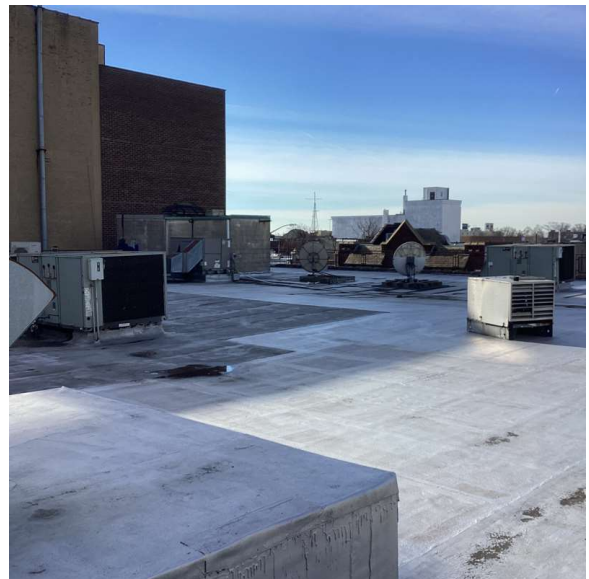
Roof 1 - Southwest view
