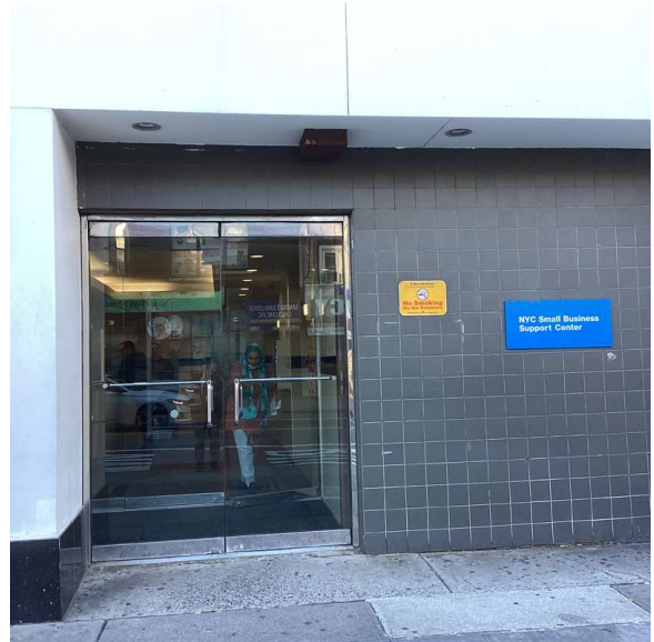
Facade A - Sutphin Boulevard
