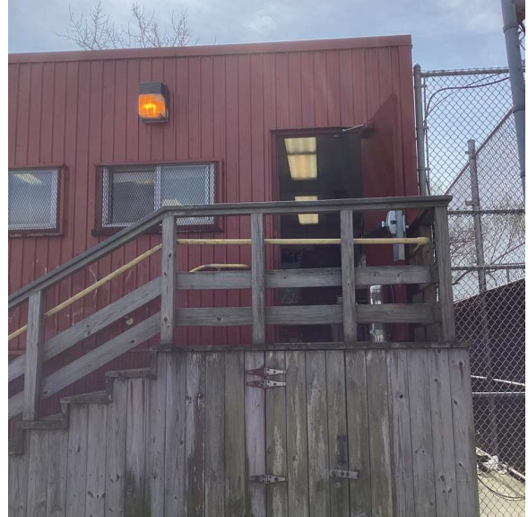
Facade A - Unit T1
