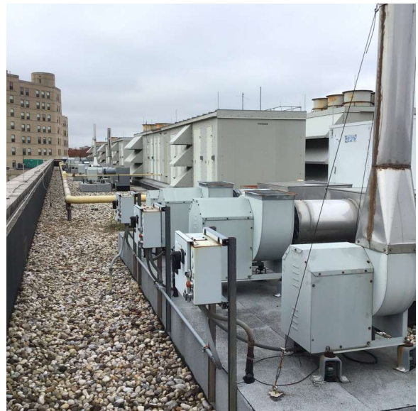
Roof 1 - Southwest view
