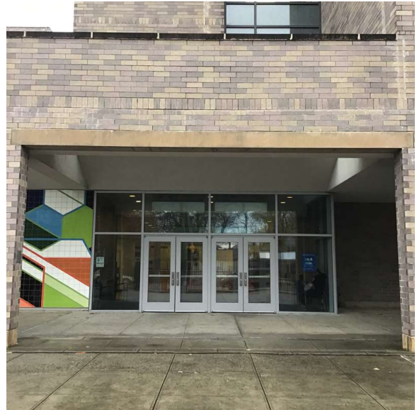
Facade A - Goethals Avenue
