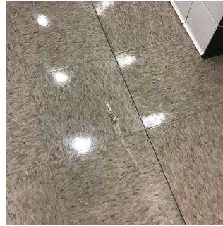
Corridor near room 121A
