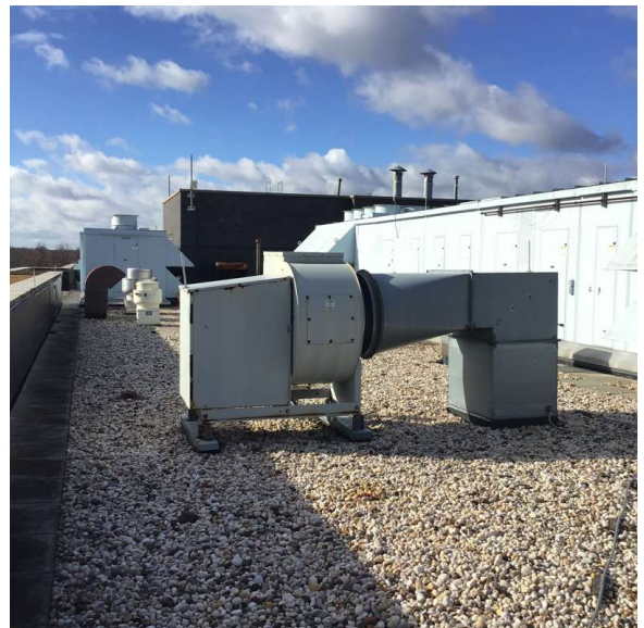
Roof 1 - Southwest view
