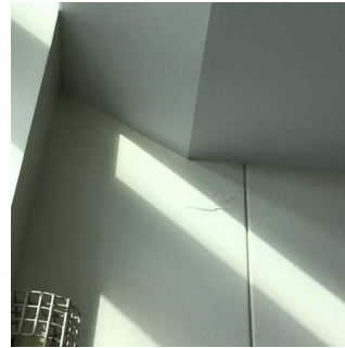
Corridor near stair A/5
