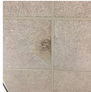
Roof 1 - Room 418, also Room 421A
