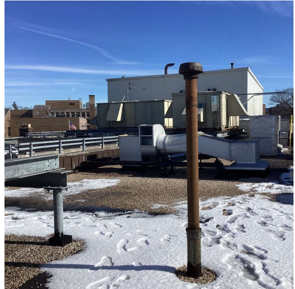
Roof 1 - Northeast view
