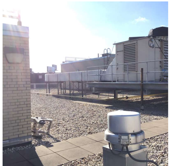
Roof 1 - North View
