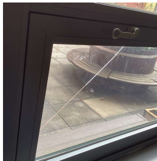
Facade H - Corridor near Room 352
