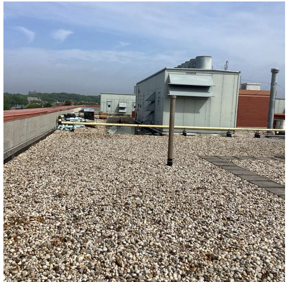
Roof 1 - North View
