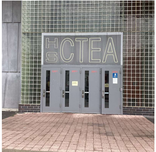
Facade A - 104th Street
