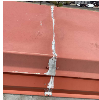
Roof 1 - Facade D
