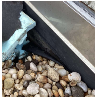
Roof 1 - Facade E
