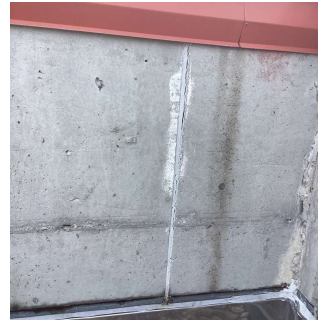
Roof 1 - Facade E
