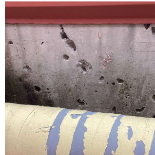
Roof 1 - Facade J
