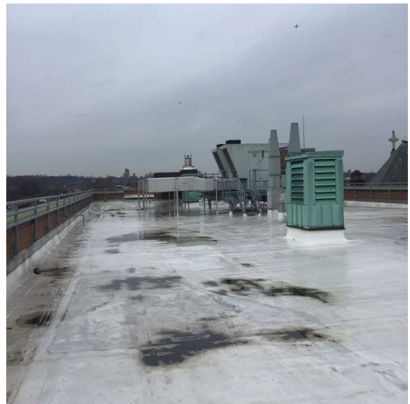
Roof 1 - North view
