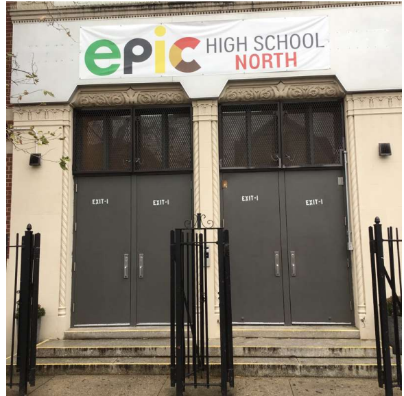
Facade A - 117th Street
