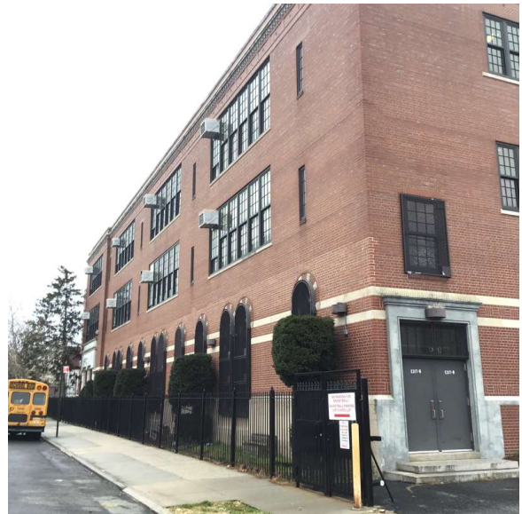
Facade A - North view
