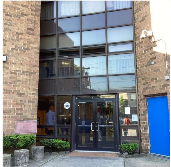
Facade A - Linden Boulevard
