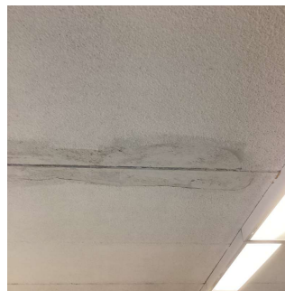
Roof 1 - Room 306, also Corridor near Room 303
