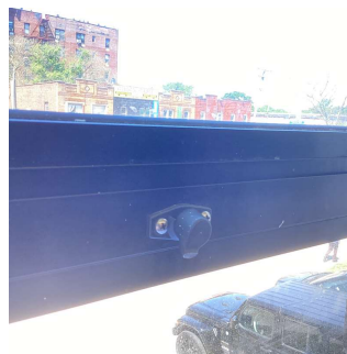
Facade F - Room 210 No violations recorded.
