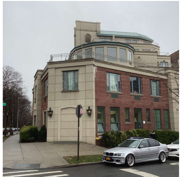
Corner of Kew Gardens Road and 83rd Drive - South view
