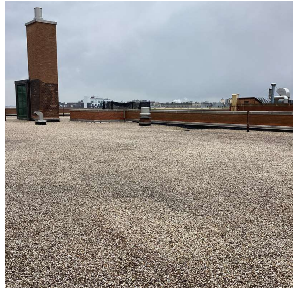
Roof 2 - Northeast View
