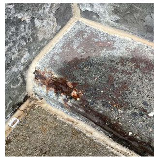
Facade H No violations recorded.
