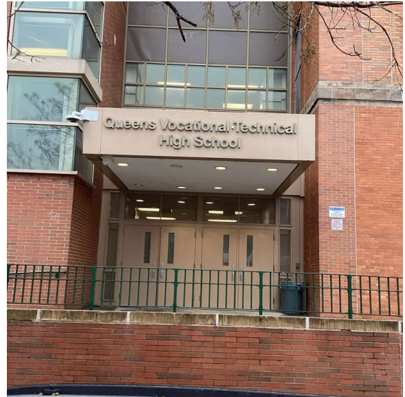
Facade A - 38th Street
